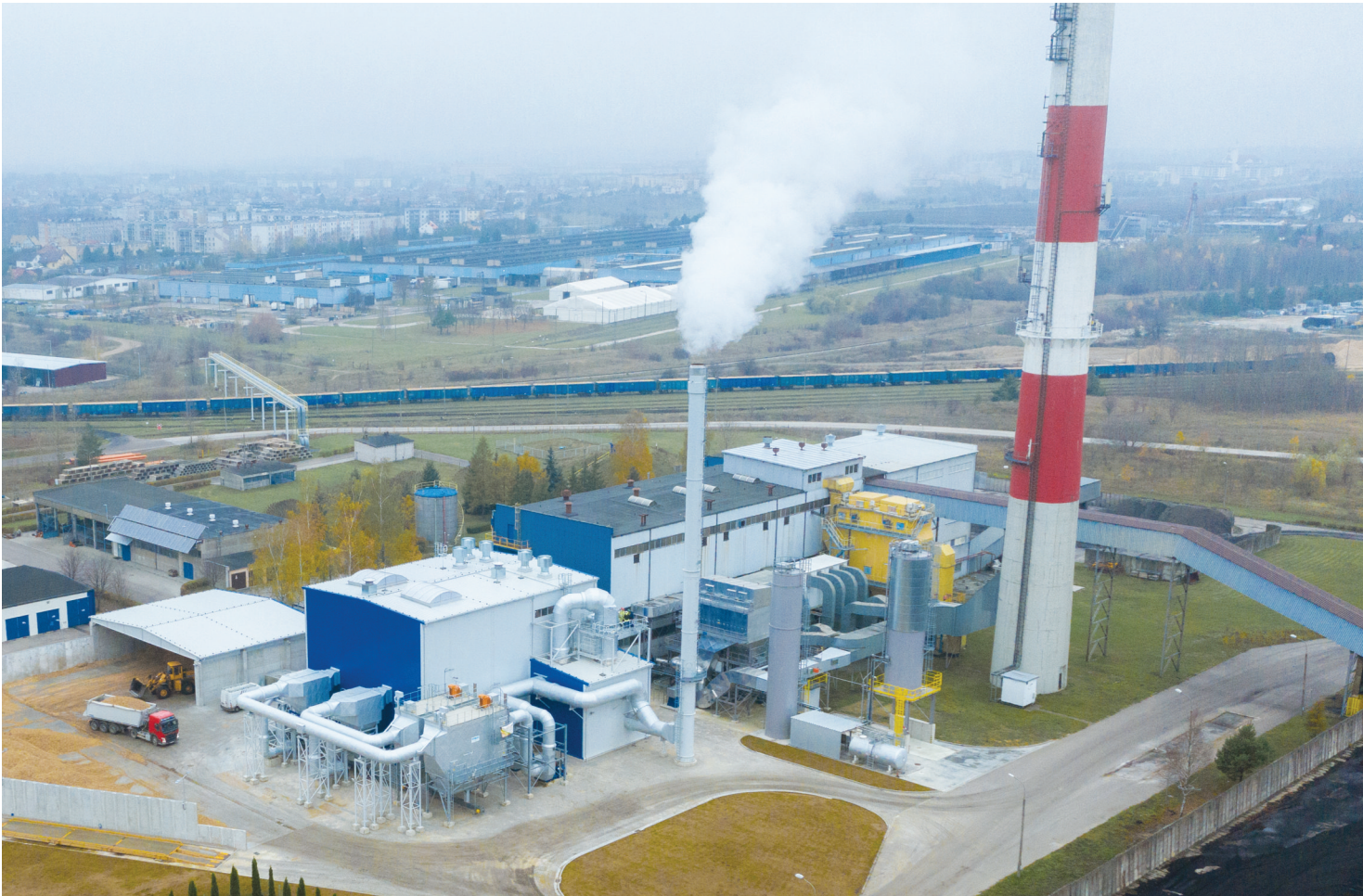
30 MW biomass boiler plant in Suwalki, Poland.
