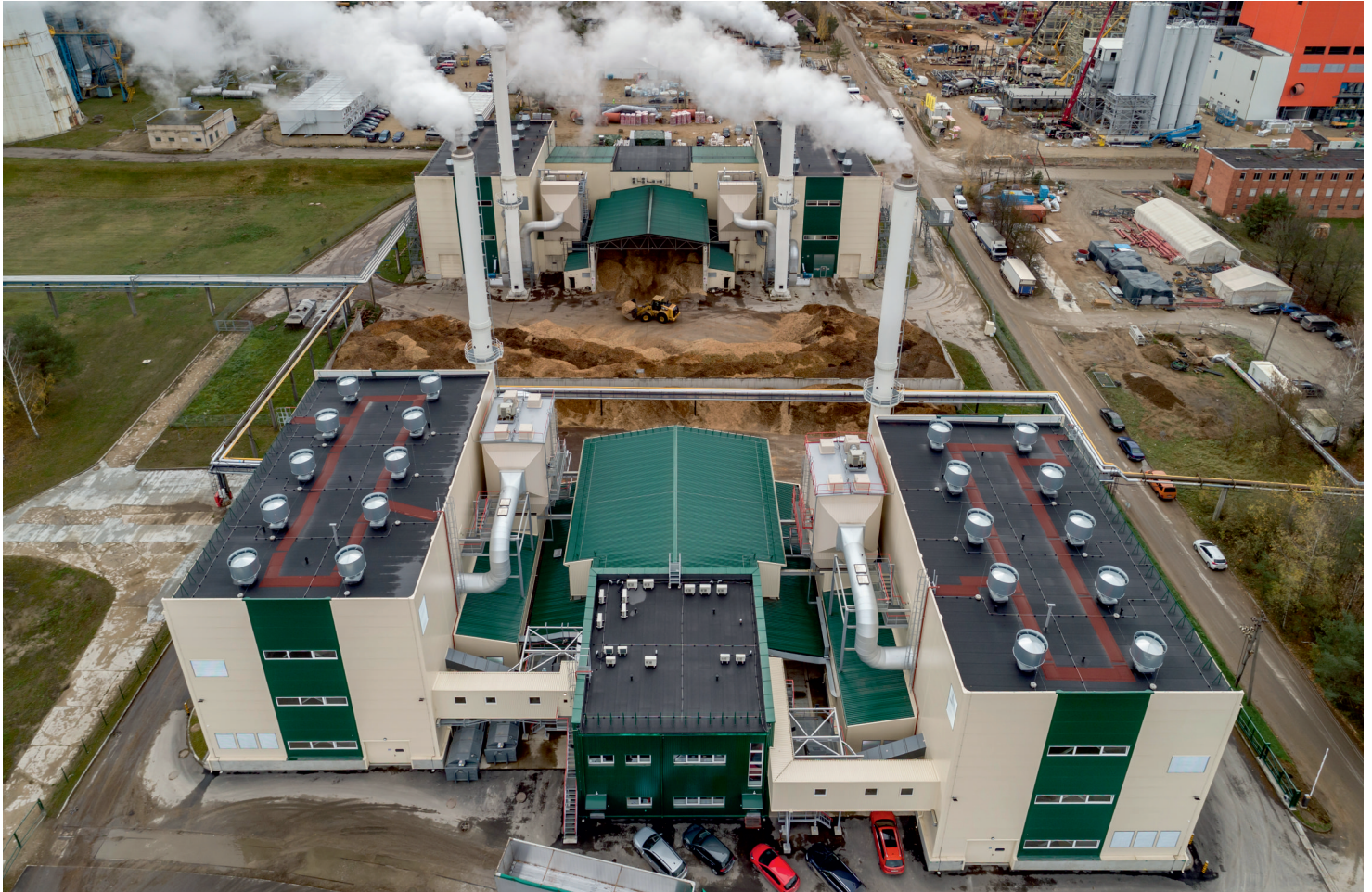
48 MW biomass boiler plant in Lithuania.
